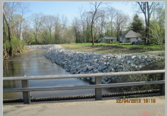
Photos are of the Feather Creek Project in Clinton, Indiana. Top photo shows project in action before it was even completed.
