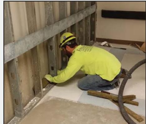
A new Post-Anesthesia Care Unit (PACU) room was successfully completed as part of Phase I. At right, a sub-contractor places fire stopping materials into an existing wall as Phase II of the surgery shutdown gets underway.
