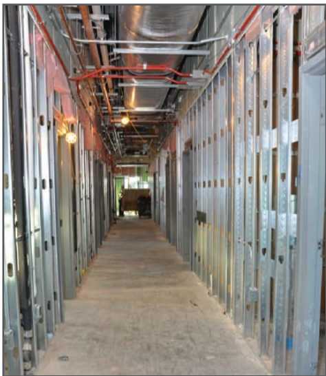
Some framing is still visible pending installation of wall insulation and drywall at the new Fort Knox Medical Clinic, which will replace the Ireland Army Medical Clinic.
