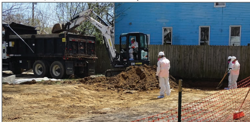
Contaminated soil is direct-loaded for transportation to a hazardous waste landfill.
