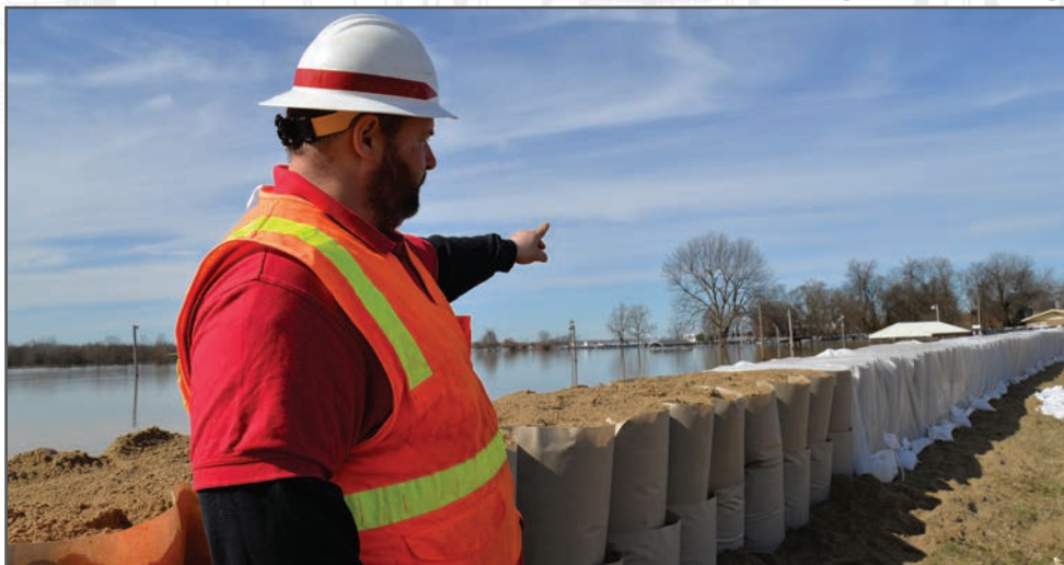
Steve Shifflett, U.S. Army Corps of Engineers Louisville District geotechnical engineer and technical lead for the Typar geocell wall in Smithland, Ky., explains the process of constructing the temporary levee Feb. 26, 2019.
