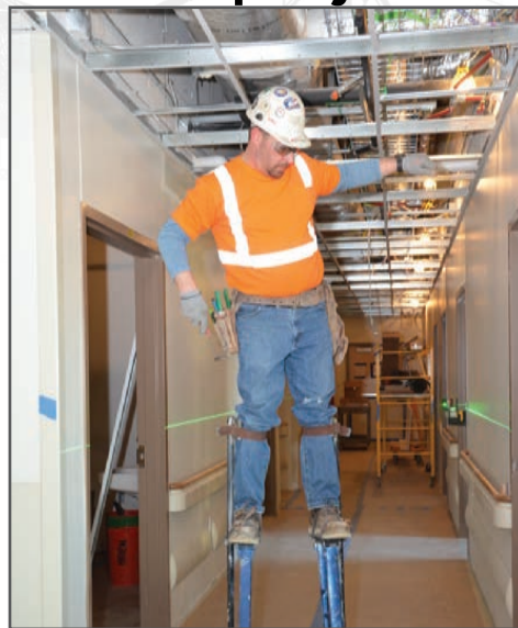
A Louisville District contractor wears stilts to assist in placing the ceiling grid of the Fort Knox Medical Clinic.
