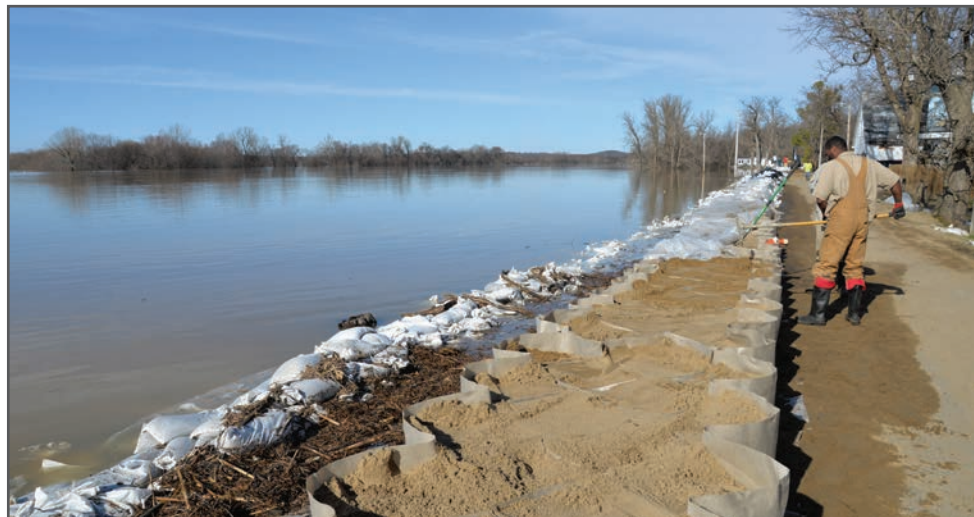
The Corps provided technical oversight on the construction of a 5,000 foot temporary levee to protect homes and businesses in the town of Smithland, Ky., during flooding in February 2019. The wall was constructed with framework made of Typar geocells and filled with loose sand. Additional sandbags were used for support.
