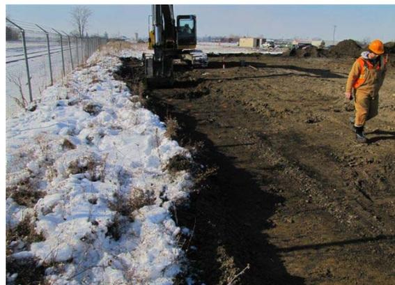
*Concrete is removed at MED-N, Coal Pile Area, to reach arsenic contaminated soil during excavation.*
