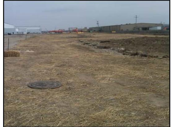
*Hay was placed on top of the backfill at MED-N, Coal Pile Area, as a temporary measure to protect the backfill. The backfill will be seeded in late spring.*
