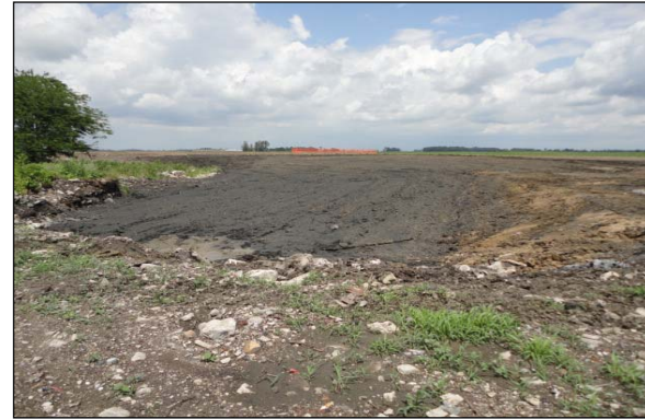
NE view, SOP-Z, Backfilled Excavation June 2013.
