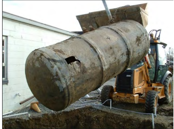
Underground Storage Tank Removal (Jacobs stock photo).
