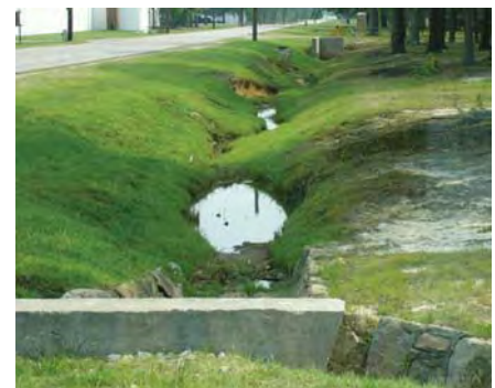
Fig.7.14 - Drainage ditches are difficult to maintain and impede mowing of the surrounding lawn areas.
