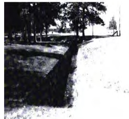
Fig. 7.12 - Where feasible, drainage ditches should be piped underground or broadened into more naturalistic swales.
