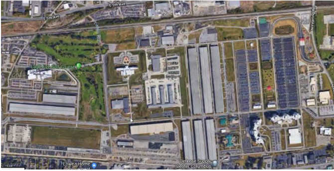
Aerial Photo of DSCC
