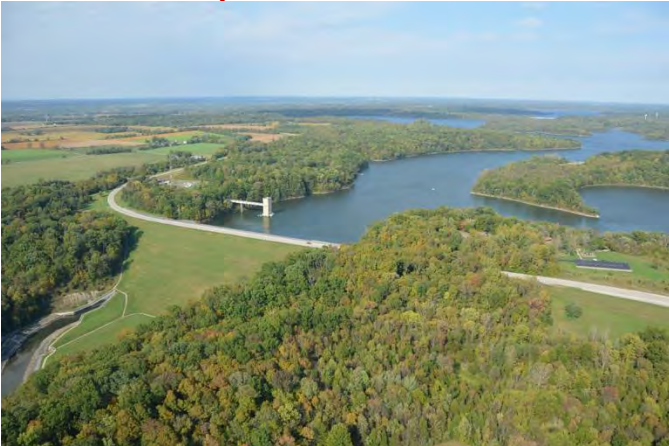
Caesar Creek Lake Dam, OH
