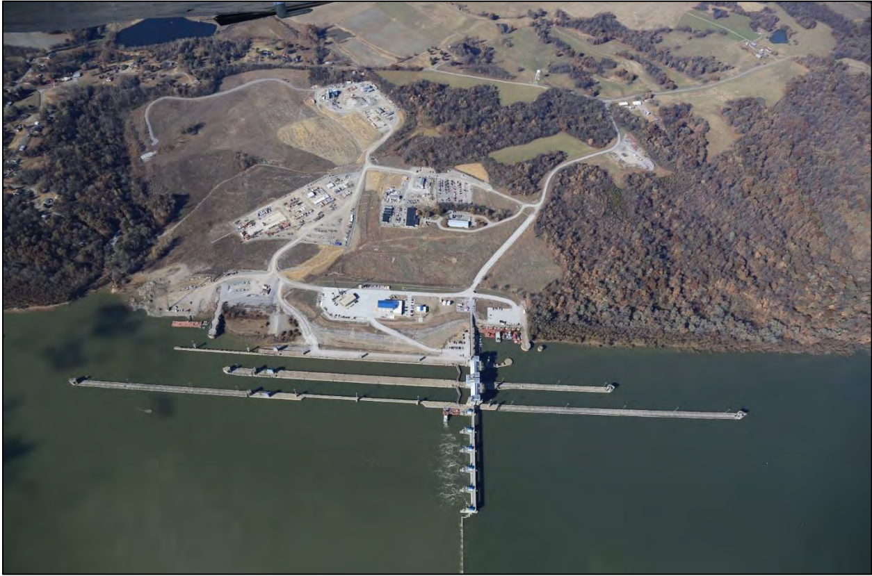
Olmsted Locks and Dam November 2019
