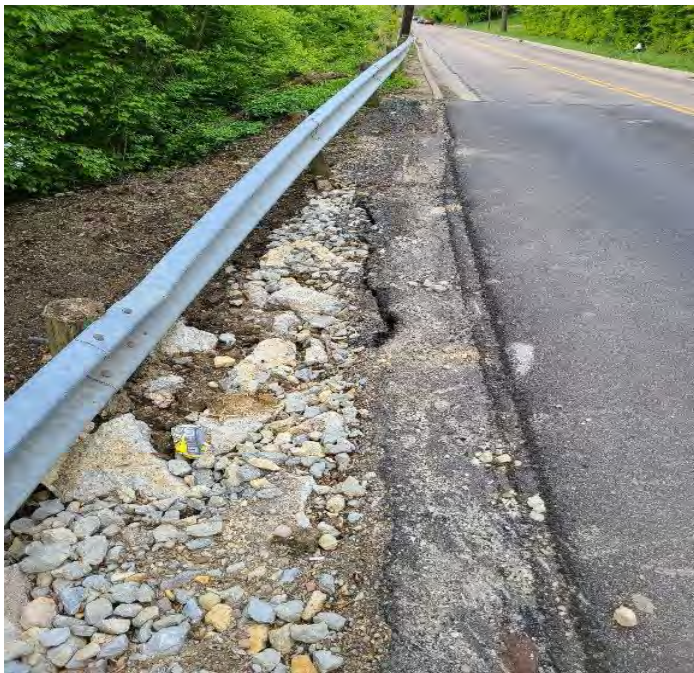
Areas of distress along E. Kemper Road affecting the roadway and guardrail
