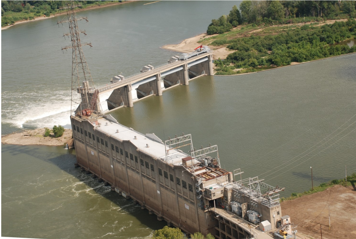
Figure 10: The hydropower station at McAlpine Locks and Dam in Louisville, KY.
