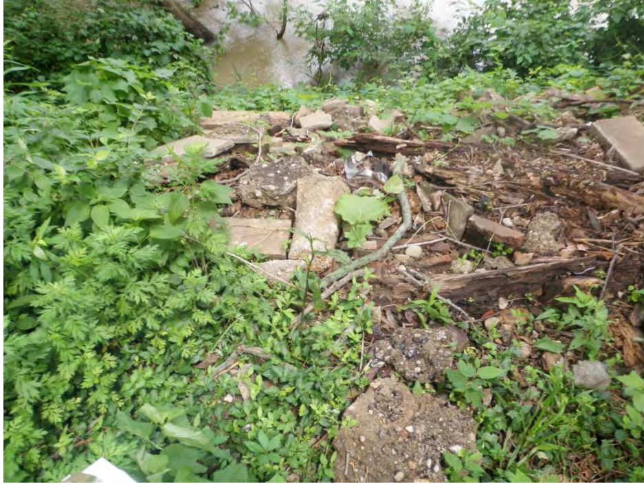
Photo 31: Debris dumped on riverward slope near Station 57+00
