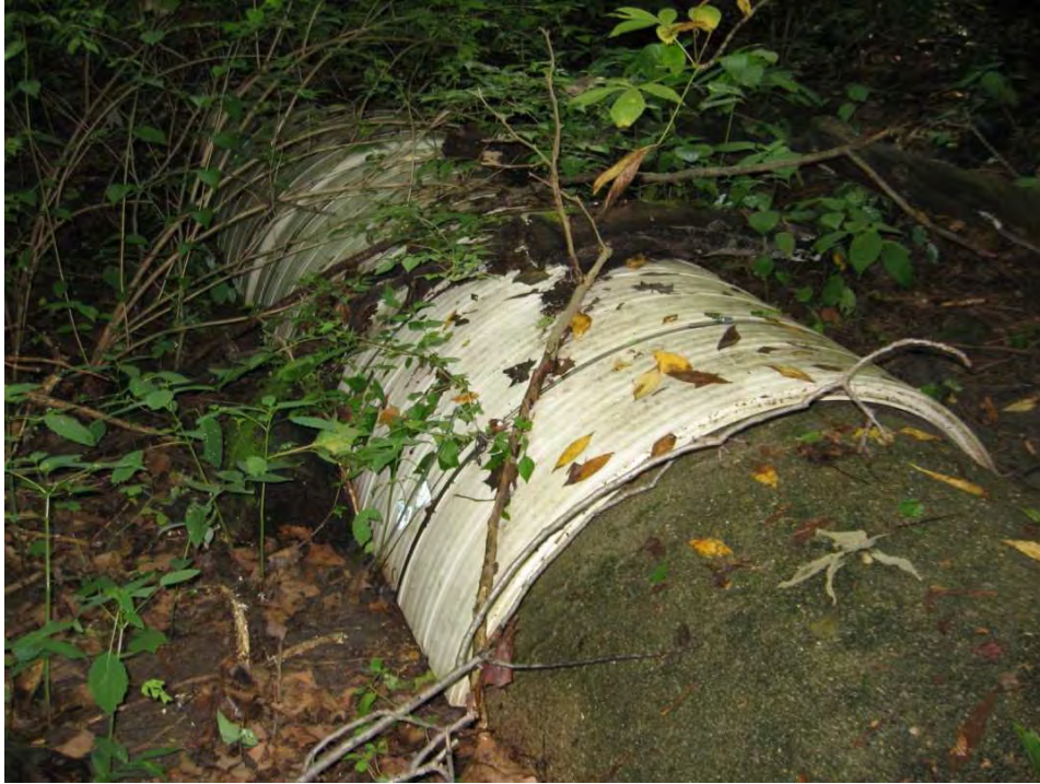
Photo 9: 36" Interceptor sewer exposed near landward toe; crosses through levee (Station 7+90)
