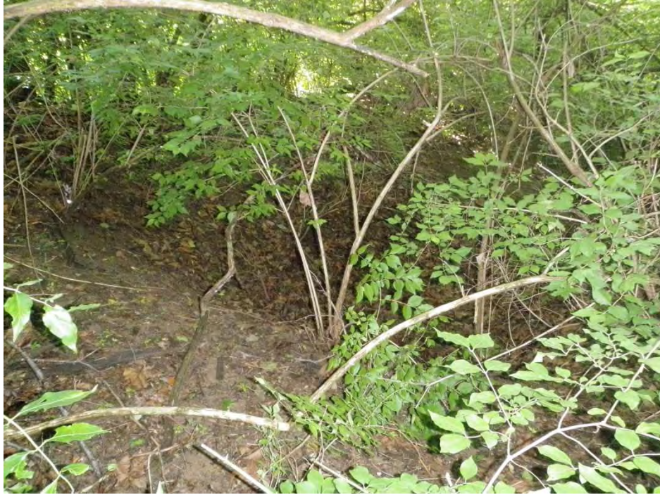
Photo 13: Large depression on riverward slope (Station 13+70) The depression is about 8-ft in diameter and 3-ft deep.
