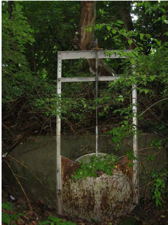
Photo 4: 48" Sluice gate on landward side of levee (Station 0+50) Note the corrosion on the gate and the large tree limb that has fallen on the guides.
