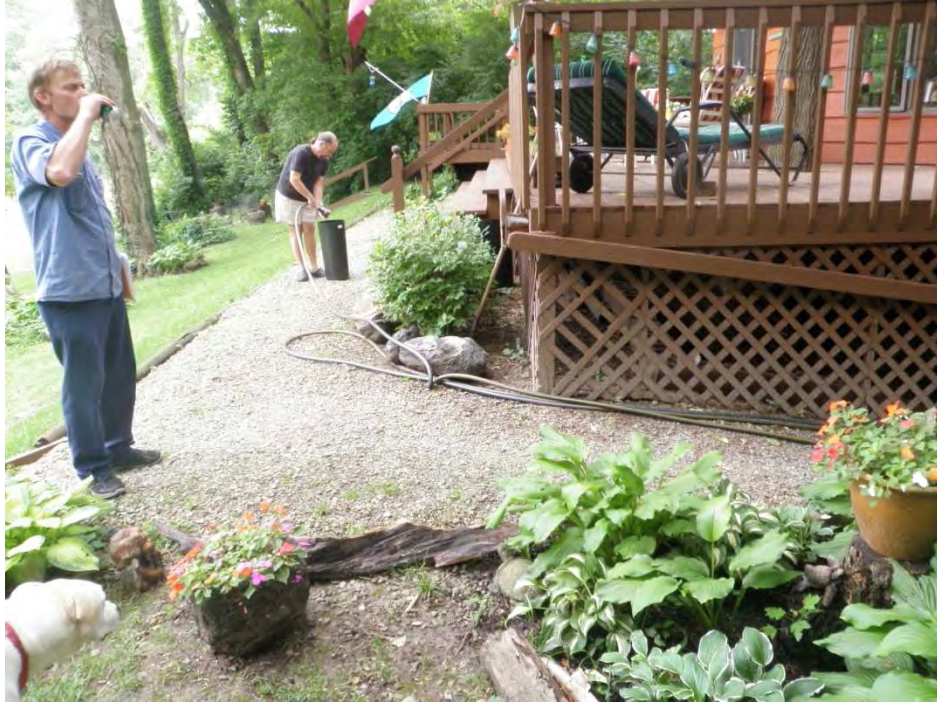
Photo 29: Deck encroaching onto levee (Station 54+00)
