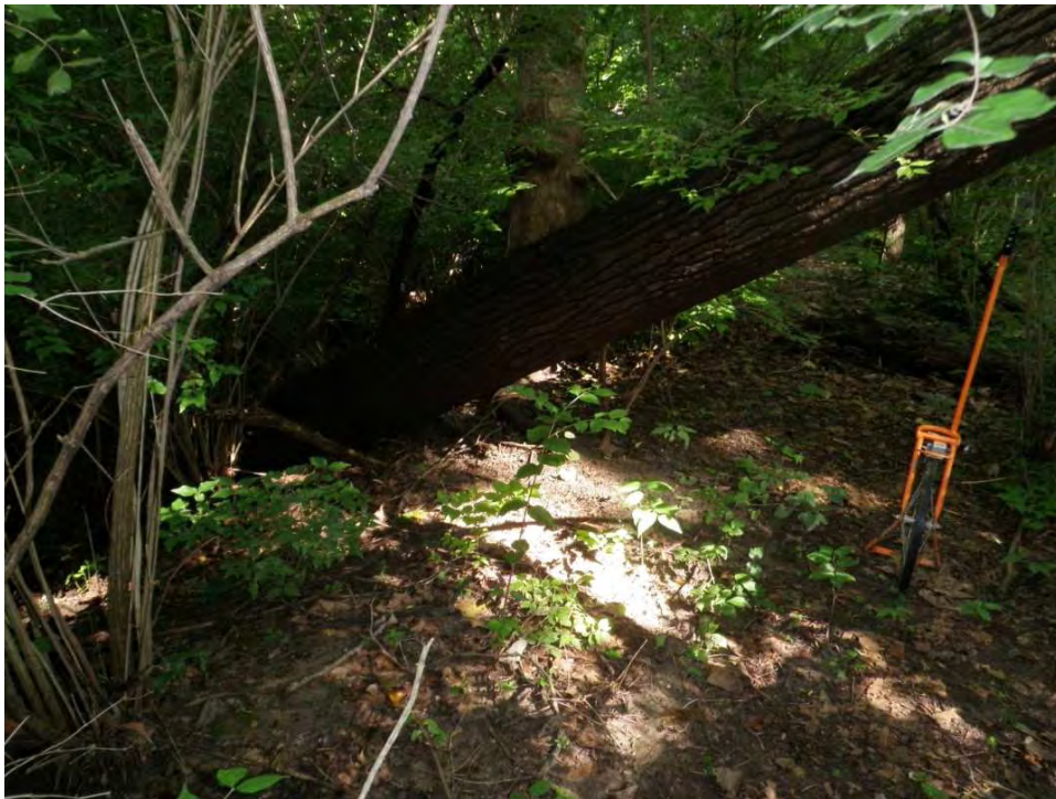
Photo 8: Large tree uprooted on levee embankment (Station 6+00)
