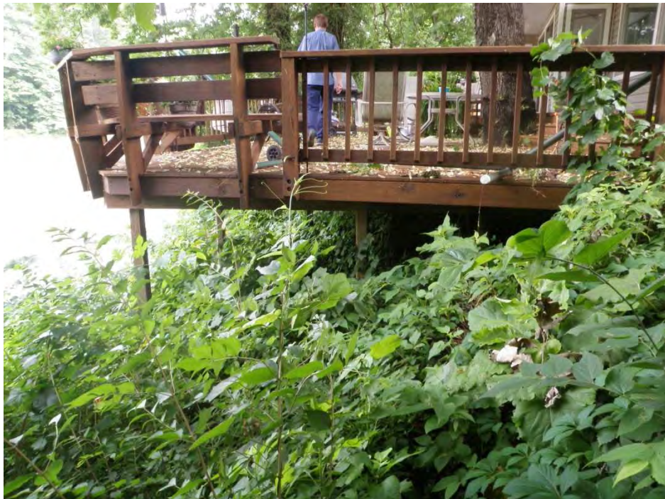
Photo 16: Deck constructed into riverward slope of levee (Station 23+90)
