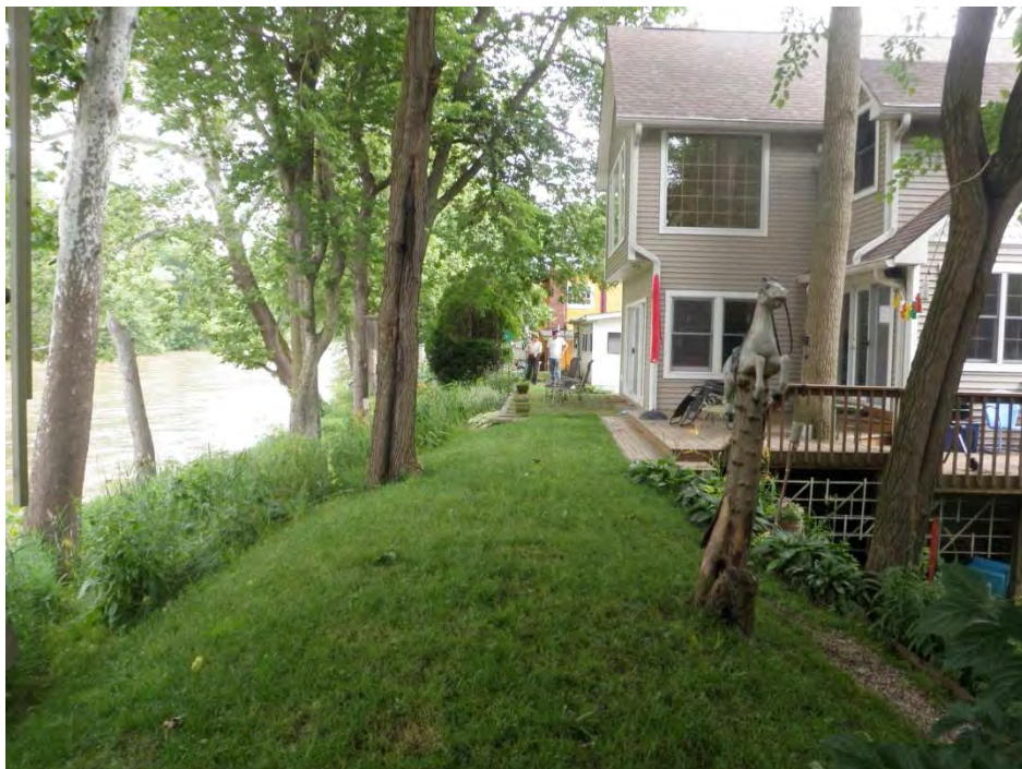
Photo 20: Riverward slope of levee and crest looking north (Station 28+00) Note the tree growth on the riverward slope and the houses encroaching onto the levee.
