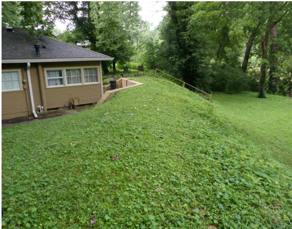
Photo 26: Retaining wall built into landward side of levee near home (Looking south near Station 46+50)
