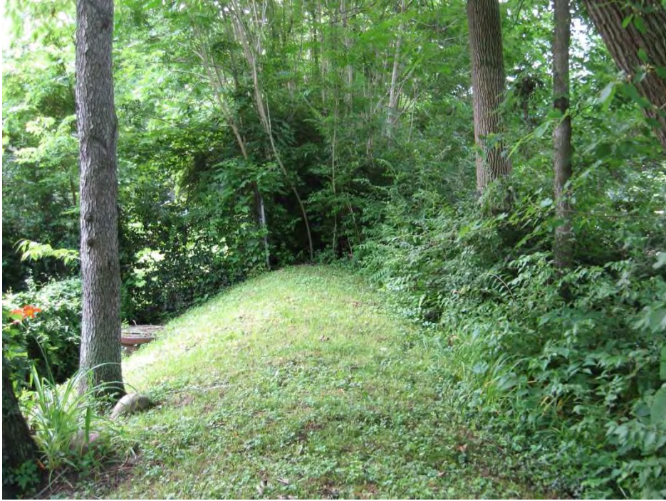
Photo 23: Crest of levee looking south (Station 36+50 +/-) Note the trees and heavy vegetative growth.
