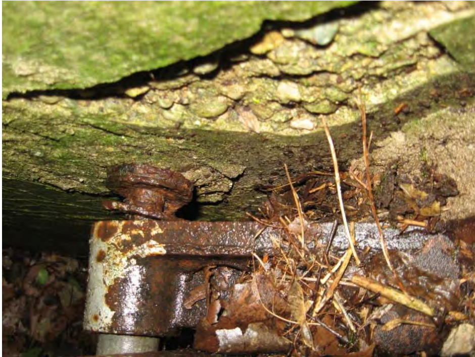
Photo 5: Corroded connections on 48" sluice gate & deteriorated headwall (Station 0+50)
