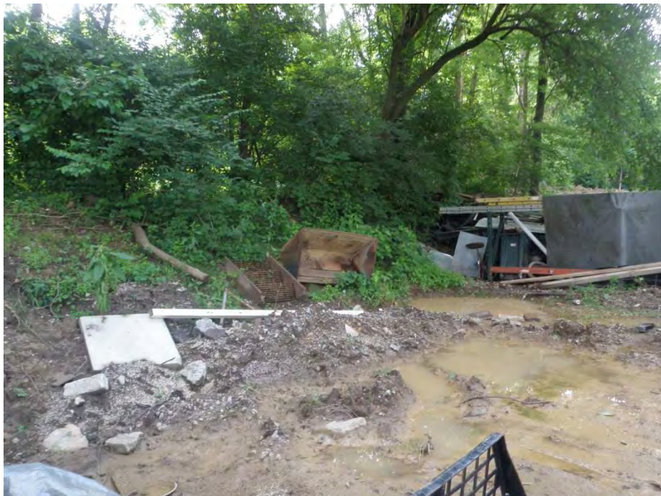
Photo 14: Encroachments and debris against riverward slope of levee (Station 17+70)
