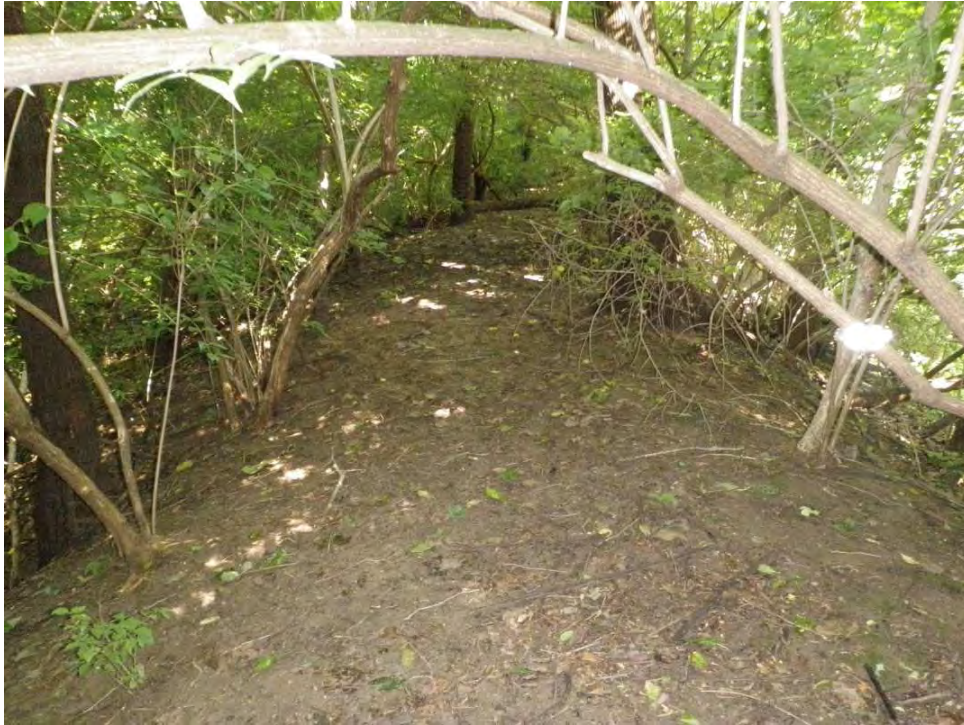
Photo 7: Levee Crest (Station 3+35) Note the extensive tree growth and lack of grass cover.
