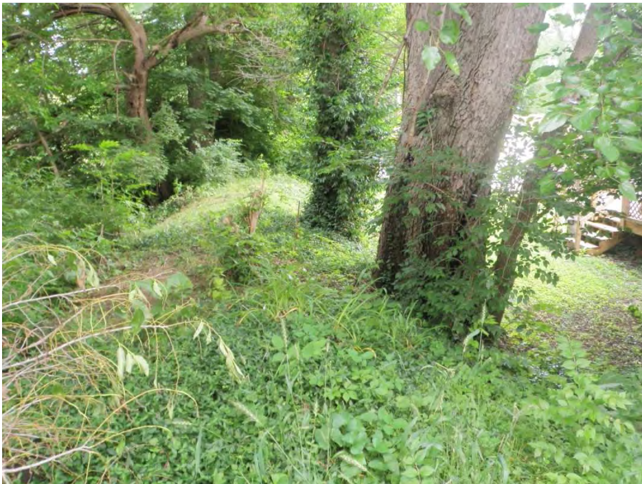
Photo 24: Crest of levee looking north (Station 36+50 +/-) Note the trees and heavy vegetative growth.
