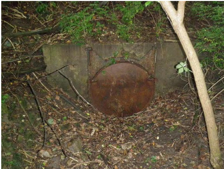
Photo 2: 48" Flap gate on riverward side of levee (Station 0+50) Note that the gate is corroded and the headwall severely deteriorated.
