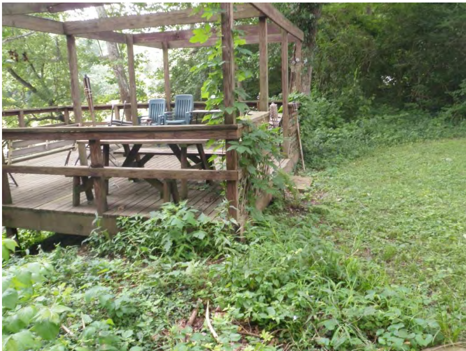
Photo 34: Deck encroaching on riverward slope of levee (Station 60+60)
