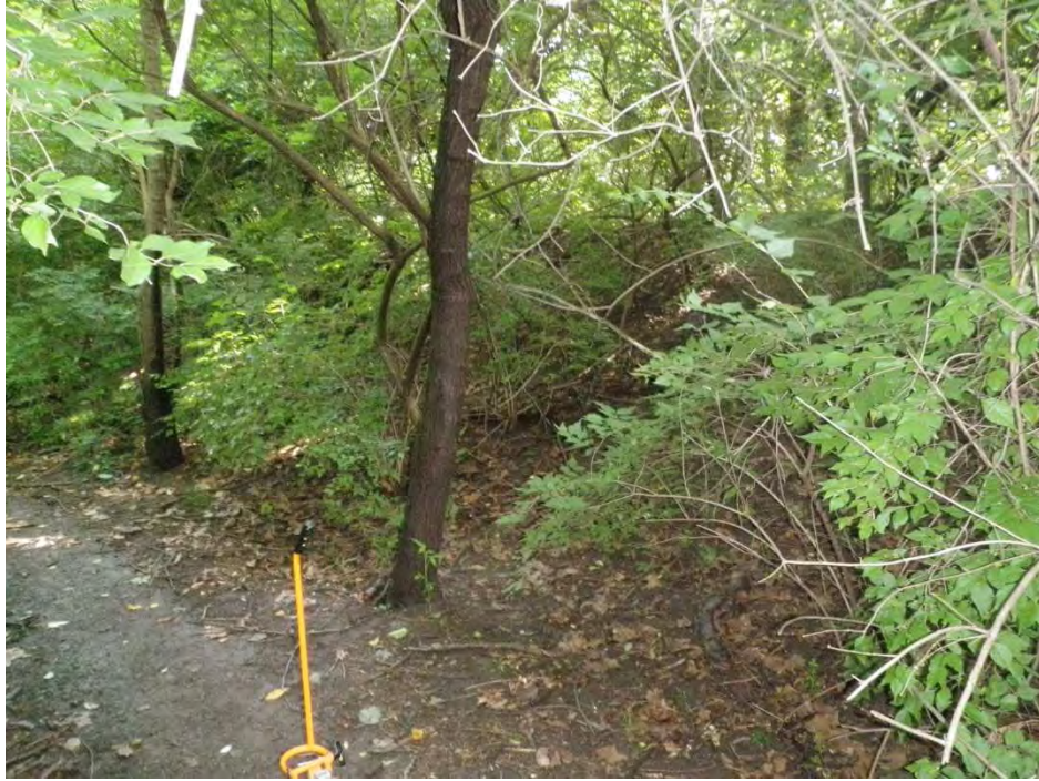
Photo 11: Riverward slope (Station 10+20) Note the extensive tree growth and lack of grass cover.
