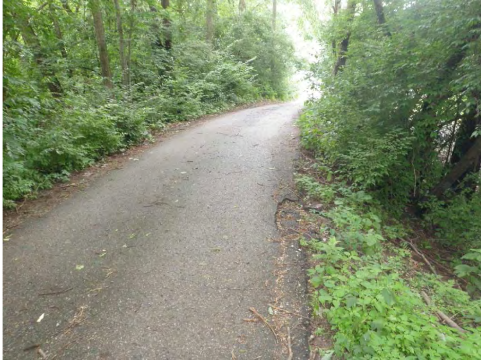
Photo 15: Riverview Drive run-up over levee at change in levee alignment (Station 22+30) Note the tree growth on the embankment slopes.
