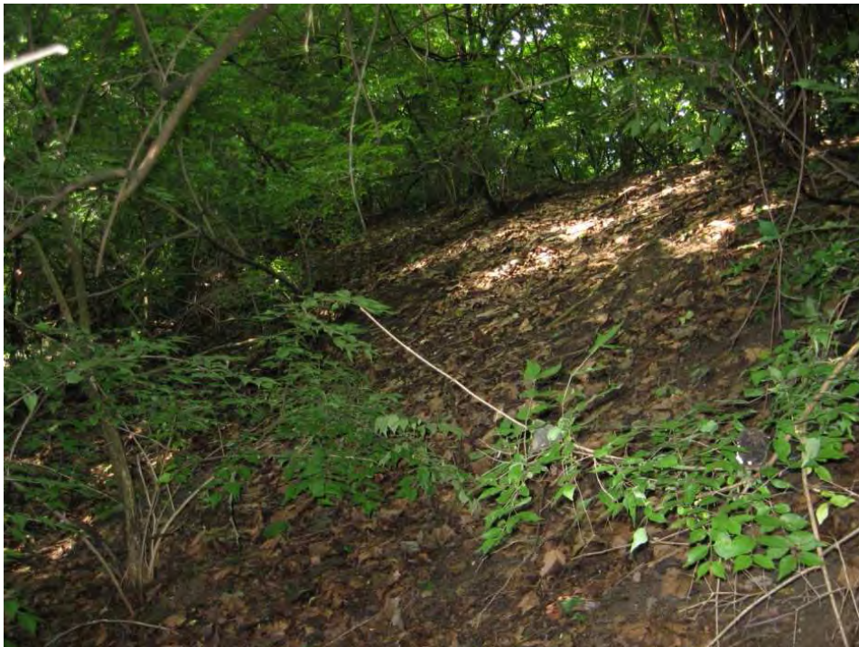
Photo 10: Landward slope (Station 9+00) Note the extensive tree growth and lack of grass cover.
