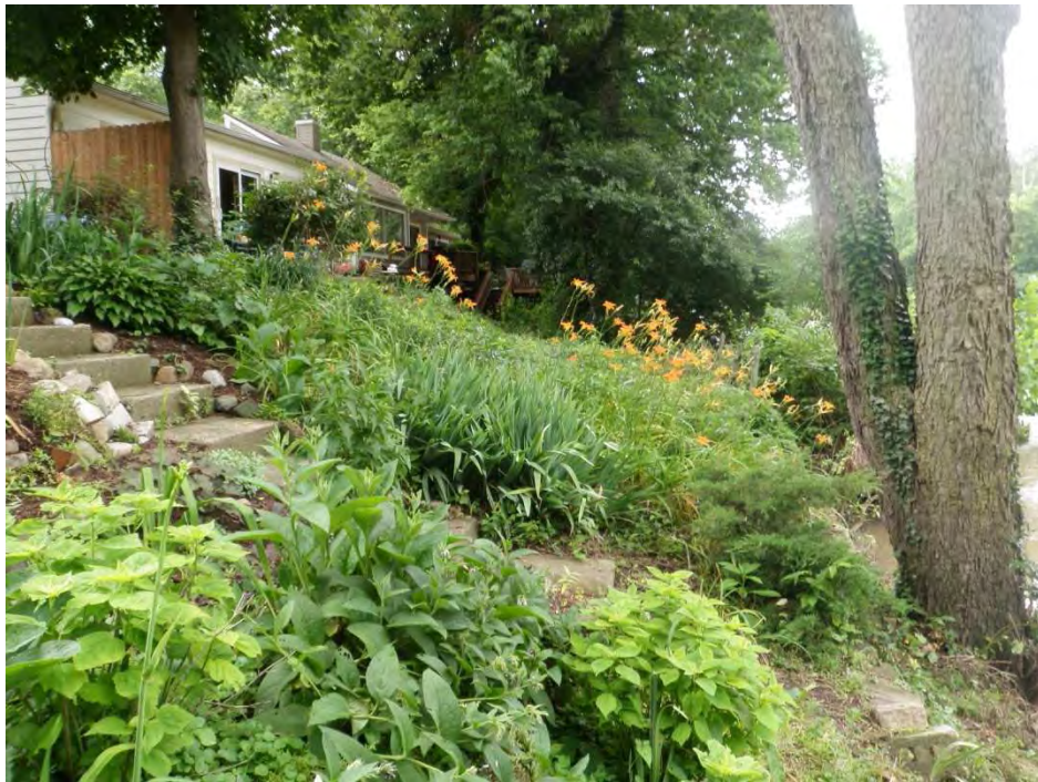
Photo 18: Riverward slope of levee looking south (Station 25+20) Note the tree growth, undesirable vegetation, and encroachments.
