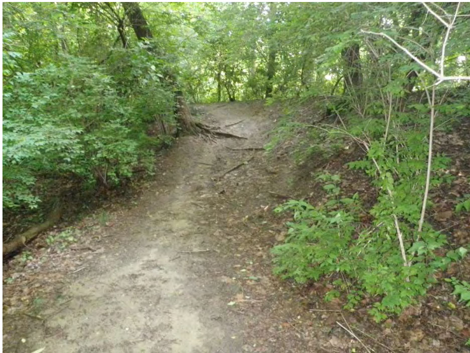
Photo 12: Trail crossing over levee, looking at the riverward slope (Station 11+30) Note the erosion and lack of grass cover.
