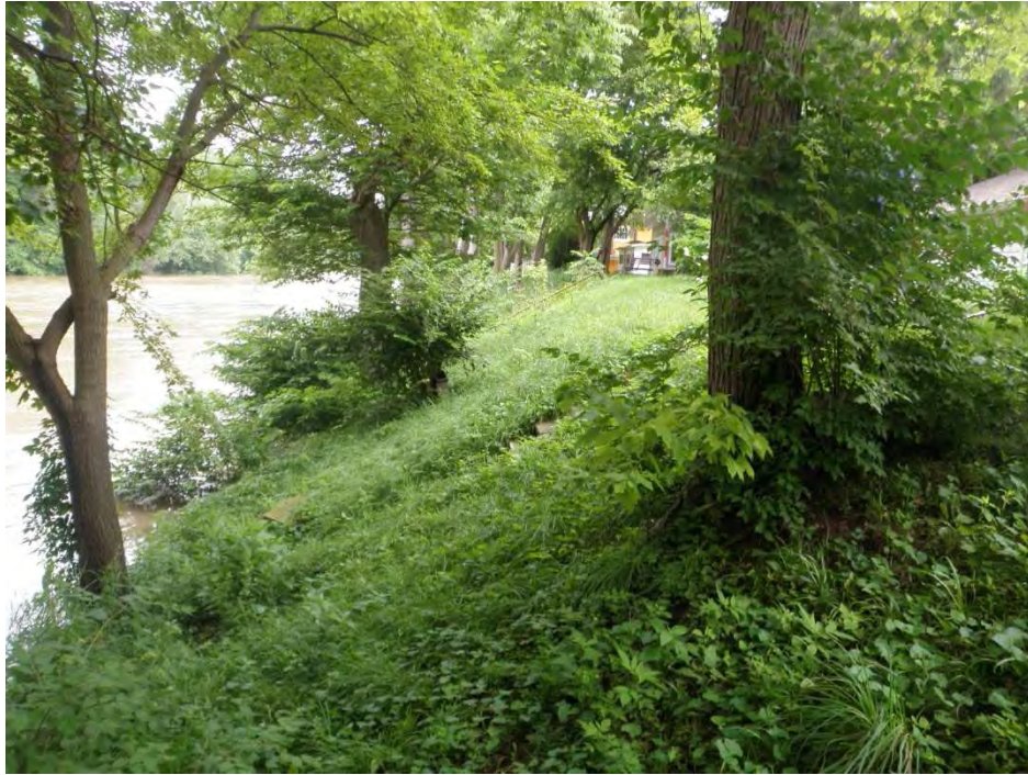
Photo 19: Riverward slope of levee looking north (Station 27+00) Note the tree growth and undesirable vegetation.
