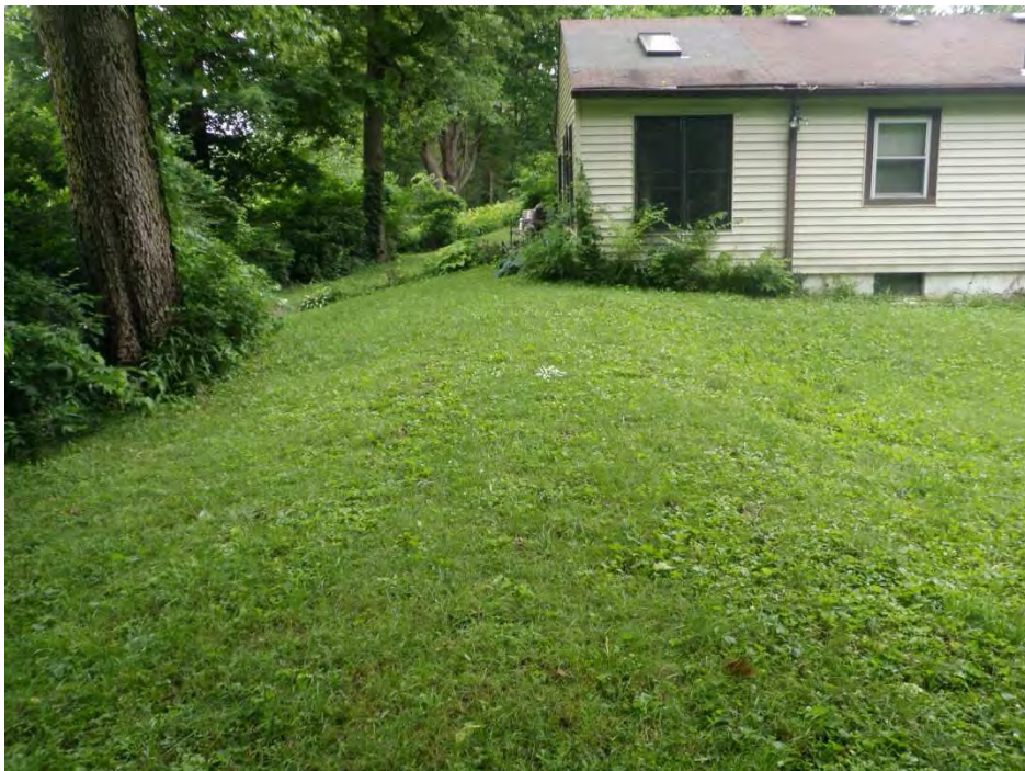
Photo 38: House with basement encroaching onto levee (looking east near Station 69+70)
