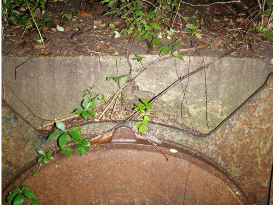
Photo 3: Concrete headwall and flap gate (Station 0+50) Note the large crack at the top of the headwall.
