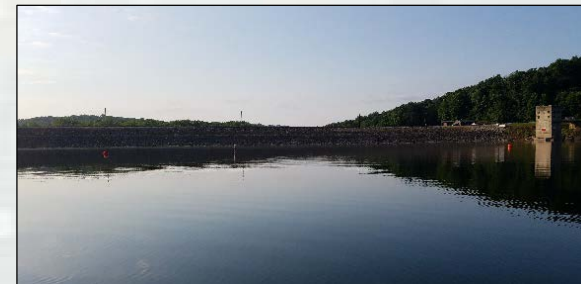
Figure 5. Monroe Lake Dam in July 2017.
